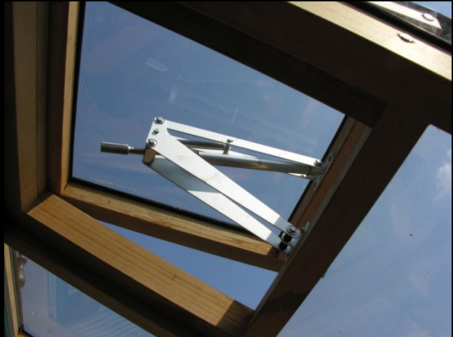
Above picture shows a triple spring autovent
